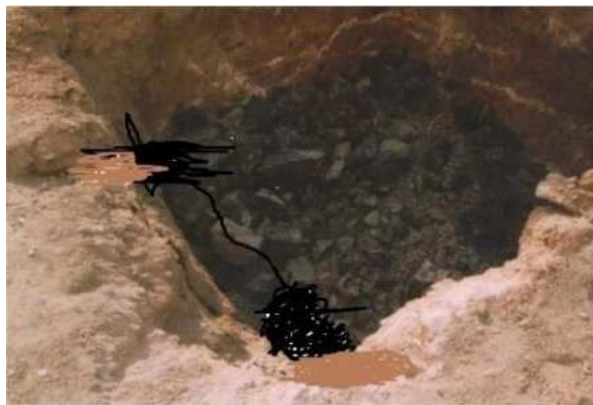
Fig - Recharge Pit of 5x5x6 feet
